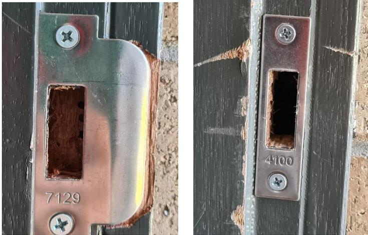
Attach the main striker plate with the screws provided and complete the lock check to ensure the door locks in both open and closed positions
